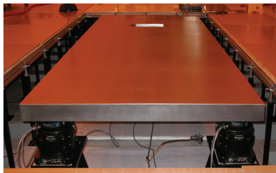
STACIS® System on “risers” installed as a custom designed TMC Quiet Island® subfloor platform to support an eBeam lithography tool in a 36 in. tall raised floor.
